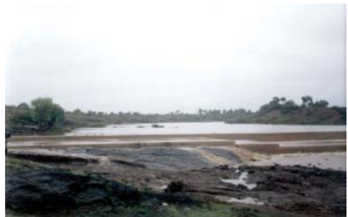
Check Dam at Sangania, Gujarat on River Malan
