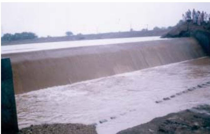
Check Dam at Dharai, Gujarat on River Bagad
