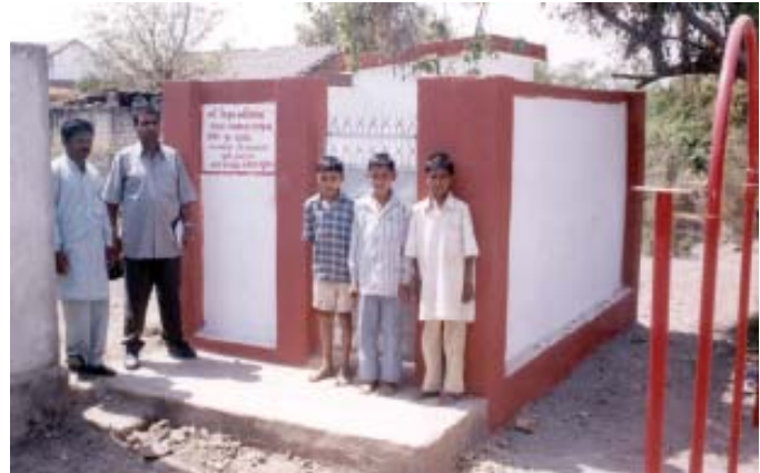
Primary school sanitation block in Dantrad village, Talaja District
